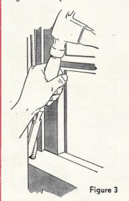
with a hammer to free further the sash from the frame as shown in Figure 3. Do this on both sides of the sash.
